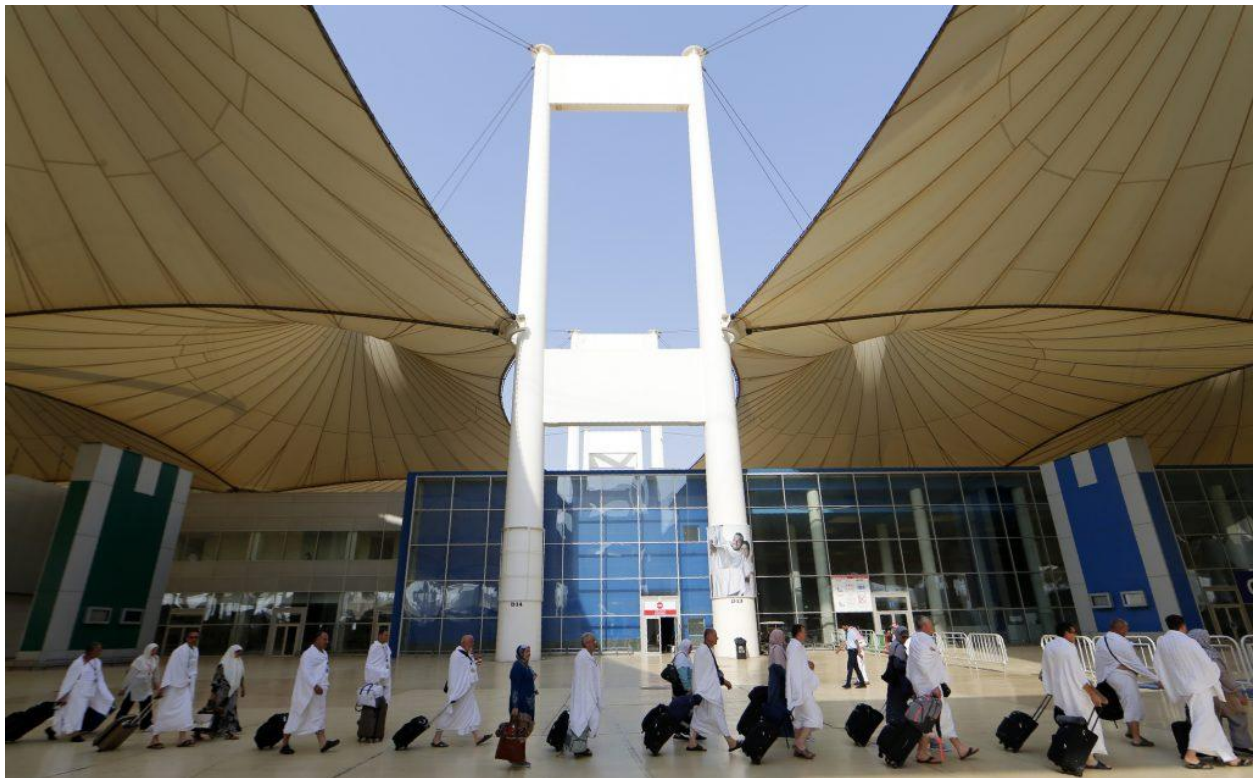
Hajj Terminal of King Abdulaziz International Airport in Jeddah, Saudi Arabia. Photo: Karim Sahib/AFP via Getty Images.
